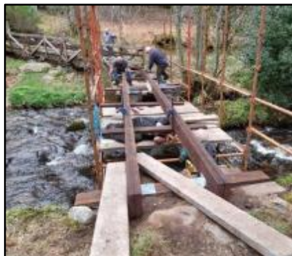
Old wood removed, new main bearers in place (left), New span finished complete with new safety wire (right)
