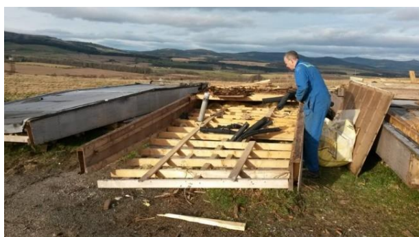
Various stages of the additional Portakabin units being stripped for materials and removed from site
