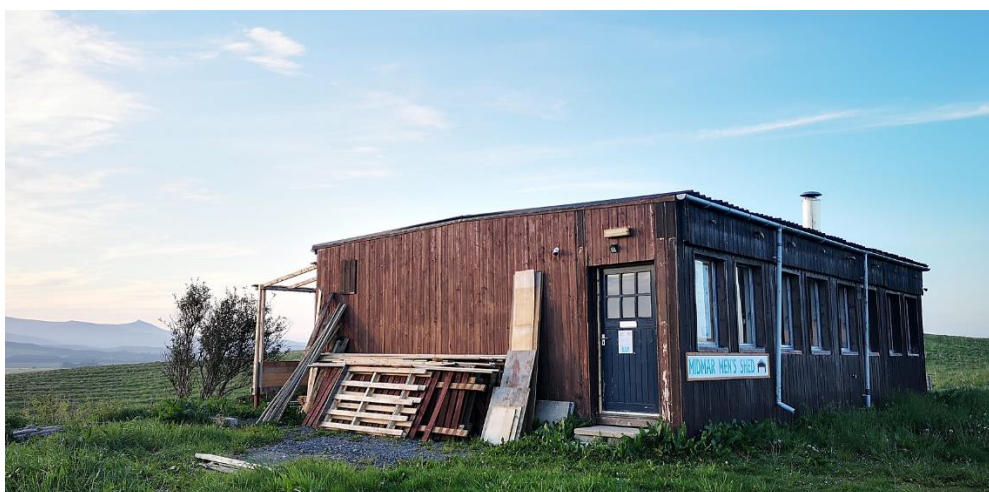
Our temporary shed with the local landmark hill Bennachie in the distance (left)
