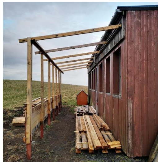
Our lean-to during construction
