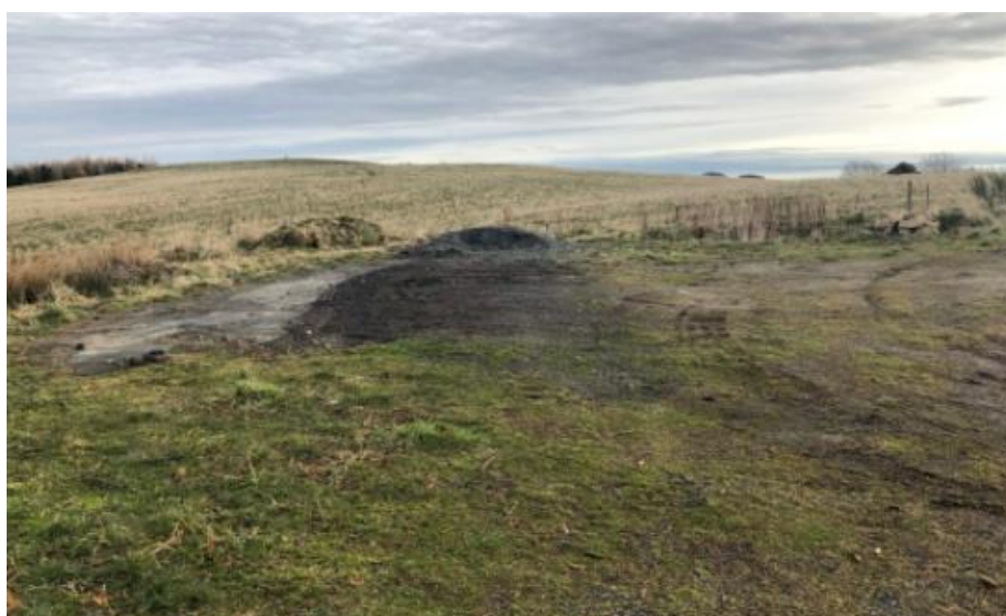
Ground-levelling prior to the arrival of the portacabin units
